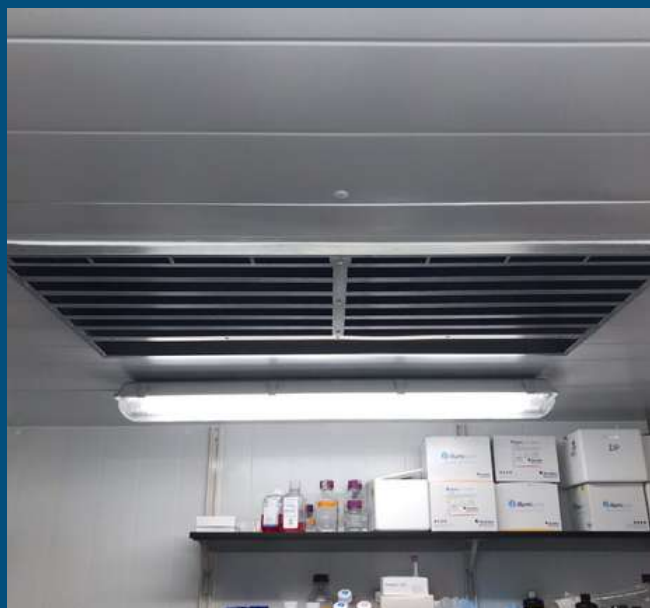
Fig. 3: LABWORKS Labtech 18-year-old environmental chamber supply and return air grill.
