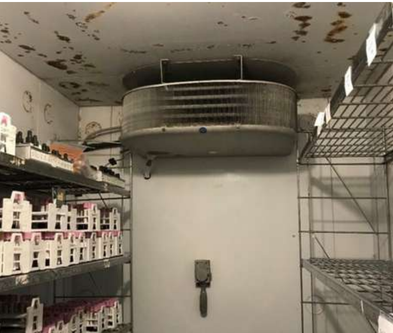
Fig. 1: Competitor's evaporator with finish damage from condensation.
